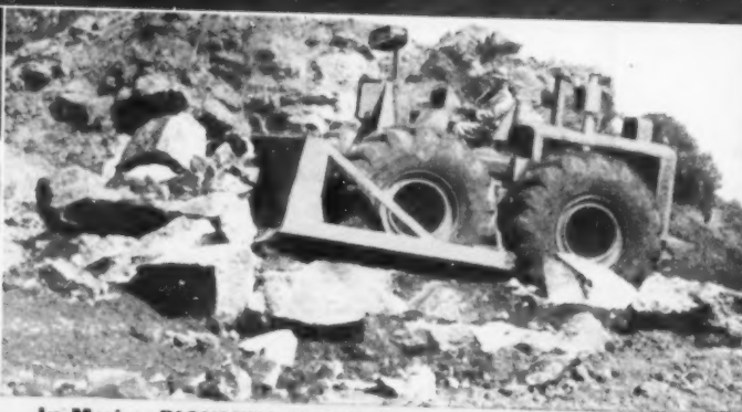
In Mexico, PIONEERS HIGHWAY —For a new super-highway connecting Mexico City and Acapulco, 6 rubber-tired Tournadozers, owned by Constructora Juarez de Mexico, S.A., are speeding initial clearing and pioneering of the rocky 5,500,000-yd. right-of-way. These 19 m.p.h. Tournadozers are removing rock, brush and stumps to smooth the grade ahead of the trucks, shovels and scrapers which are handling final excavation. Big 4-wheel air brakes (2822 sq. in. braking surface) gives operator complete safety on hills.
